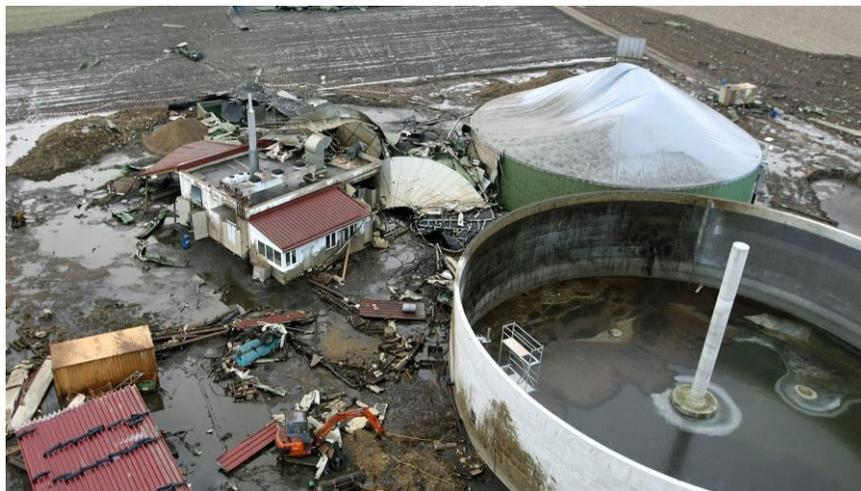
**Figure 1:** Biogas plant after explosion.
